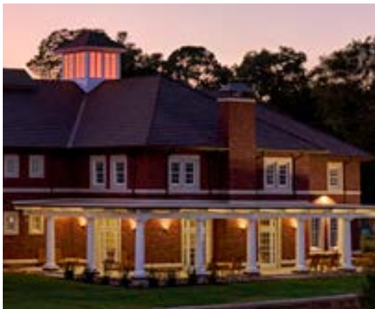
Newer facilities, like the LEED Certified Dawkins Welcome Center (shown), the LEED Gold Student Life and Technology Center, and the Miller Creative Quad, stand alongside historic buildings that carry the legacy of Hendrix while serving present needs.
